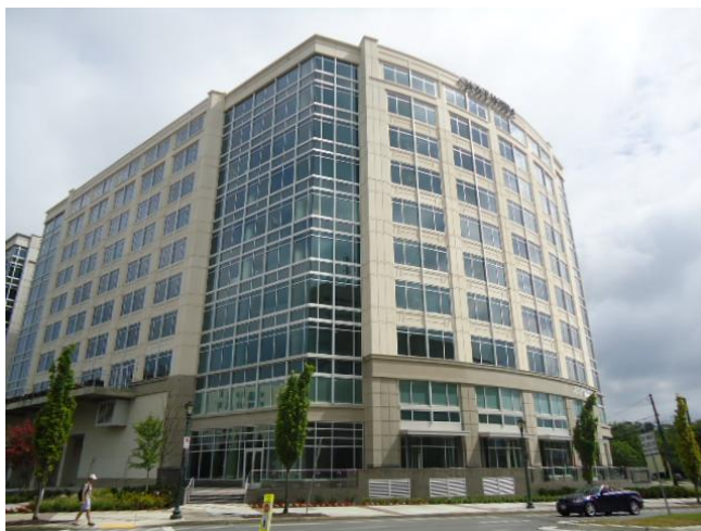
Figure F.4: South West Corner – by JMV
